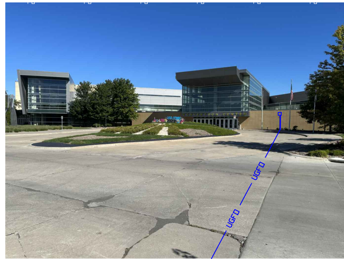
10 PHOTO - FIBER ROUTE VIEW: LOOKING NORTHWEST
