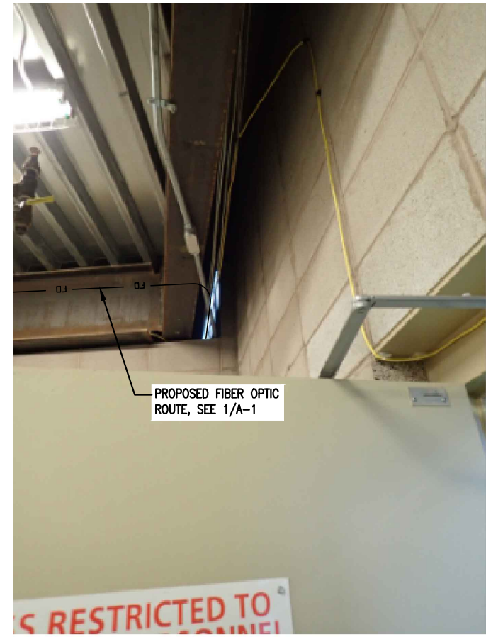
7 PHOTO - FIBER ROUTE VIEW: LOOKING NORTH
