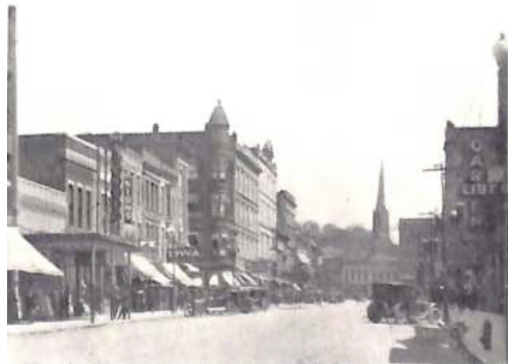
Figure 2: 500 Block of Broadway in 1921. The four bays are on the left side in the middle. Courtesy of Richard Warner and Pottawattamie County Historical Society (PCHS).
