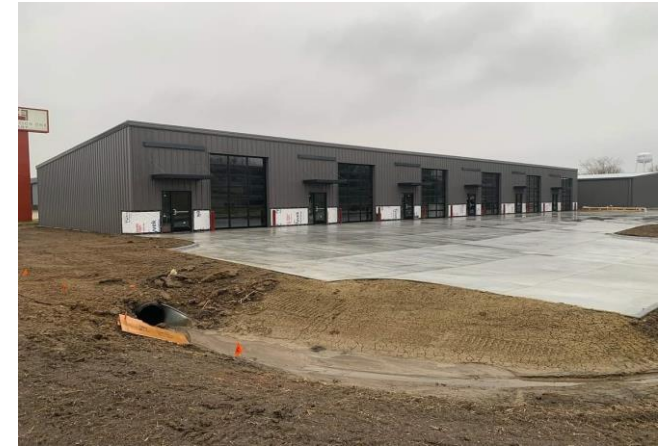
Flex Space Building Examples
