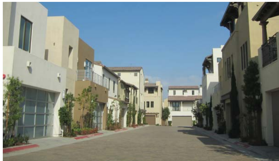
Townhomes with tuck-under garages
