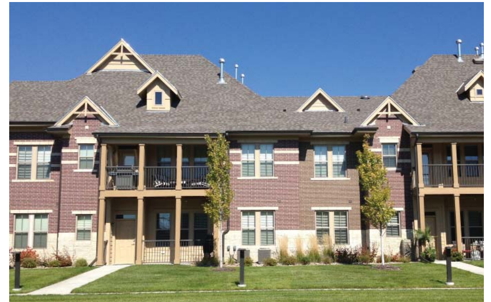
Two and three story apartment building with rear tuck-under parking
