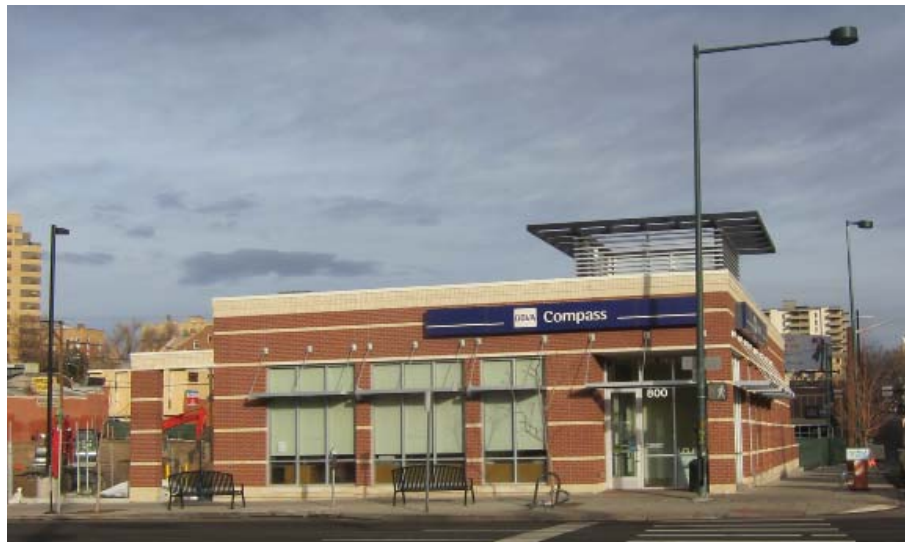
One-story stand-alone retail building
