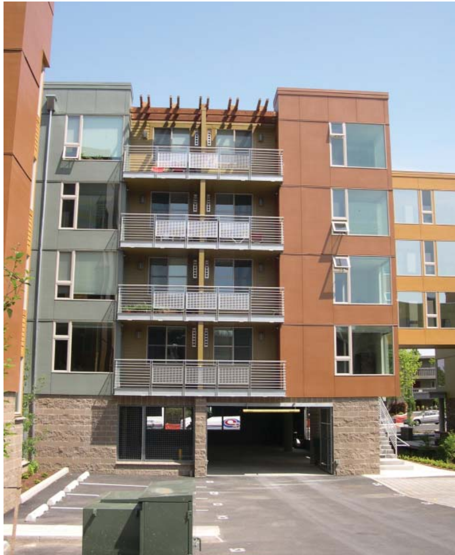
Apartment building with internal parking pedestal
