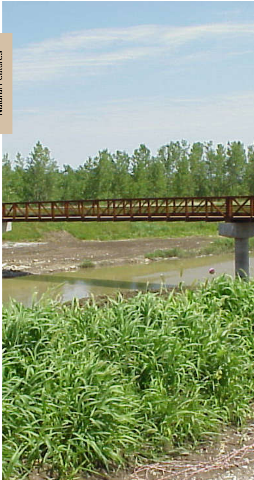
INDIAN CREEK TRAIL BRIDGE
