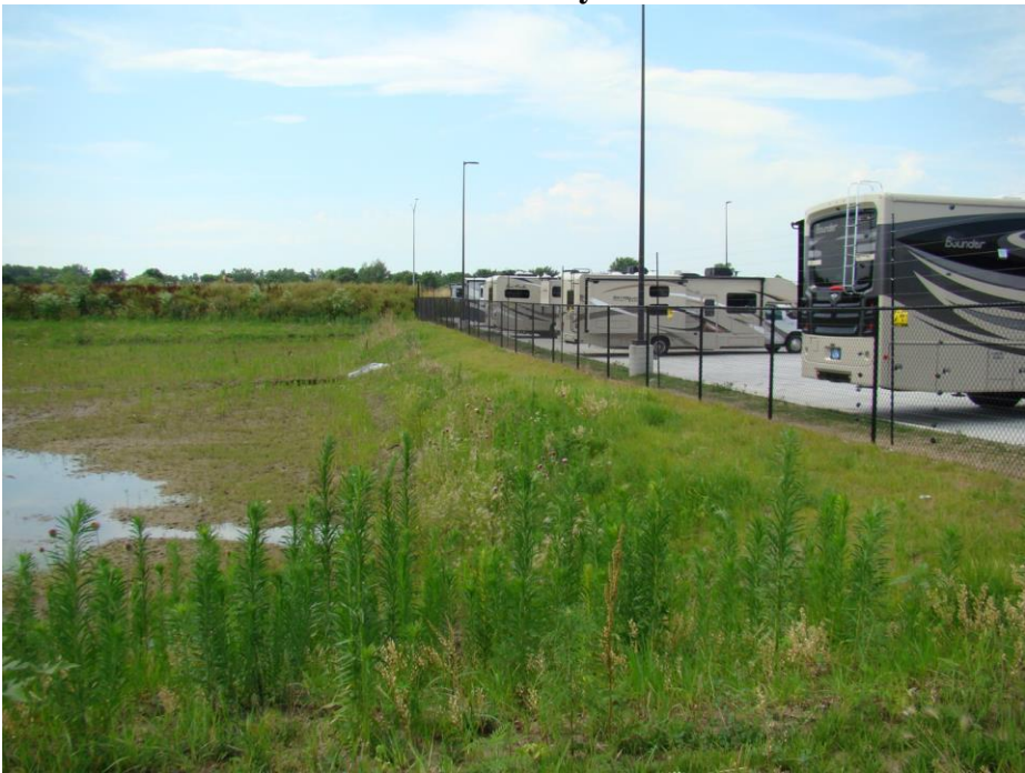
Exhibit B: View of the electric security fence that faces the residential area to the east.
