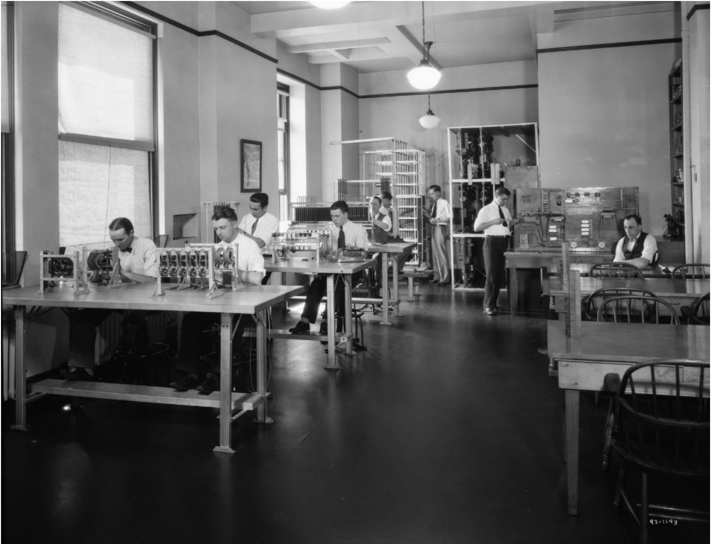
Figure 11: This photograph is included as an example of what telephone exchanges generally looked like on the interior. This photograph was NOT taken in the 12 Scott Street facility. It was taken at an unknown location and is titled, "A group of men working on some telephone equipment in a workshop." The photograph illustrates repair space at a typical Northwestern Bell Telephone Company facility and the finishes within the rooms where the engineers typically worked. A past employee of the Council Bluffs exchange at 12 Scott Street remembered the space on first floor being similar to this in the 1950s: open with work desks. Photographic source: Bostwick-Frohardt Collection, Owned by KM3TV and on permanent loan to The Durham Museum. Identifier BF92-1143. Dated 1931-04-29.
