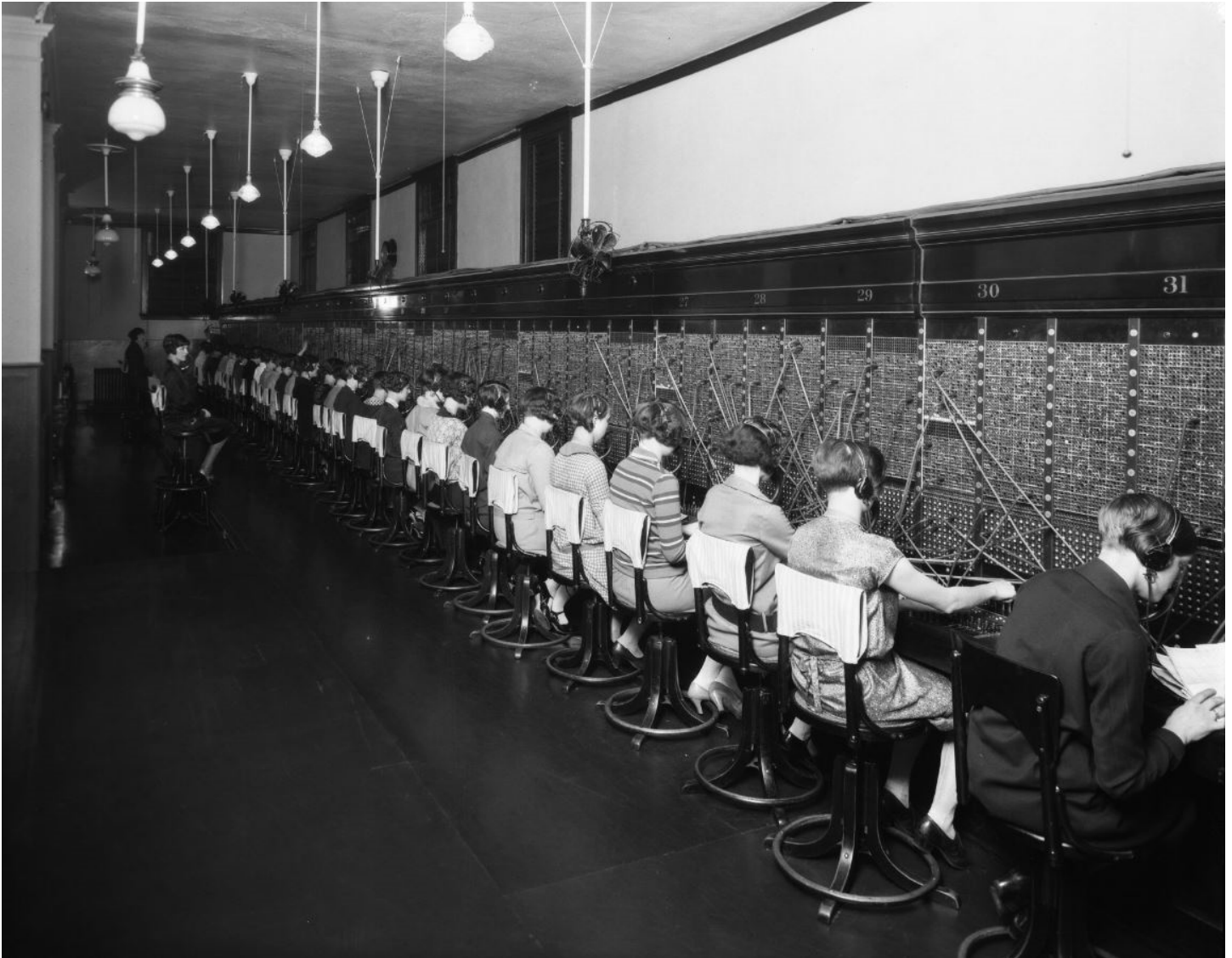
Figure 8: This photograph is included as an example of what telephone exchanges generally looked like on the interior. The switchboard equipment and switchboard operators shown here would be an important part of a typical Northwestern Bell Telephone Company facility such as the exchange at 12 Scott Street. The photograph illustrates the types of interior finish materials used in rooms where the switchboard and switchboard operators were located. Equipment and staff like this occupied the second floor on the east half of the building at 12 Scott Street. The photograph is captioned "Telephone operators working the switchboard at the Council Bluffs, Iowa exchange," and is a part of the Bostwick-Frohardt collection. Although labeled as the Council Bluffs office, this is NOT the 12 Scott Street location. The window fenestration on the right-hand side and in the background of the photograph does not appear to match the existing building. In addition to spacing and lack of grouped window compositions, each of these openings appear to have a transom above. Photographic source: Bostwick-Frohardt Collection, Owned by KM3TV and on permanent loan to The Durham Museum. Identifier BF92-686. Dated 1921-12-18.
