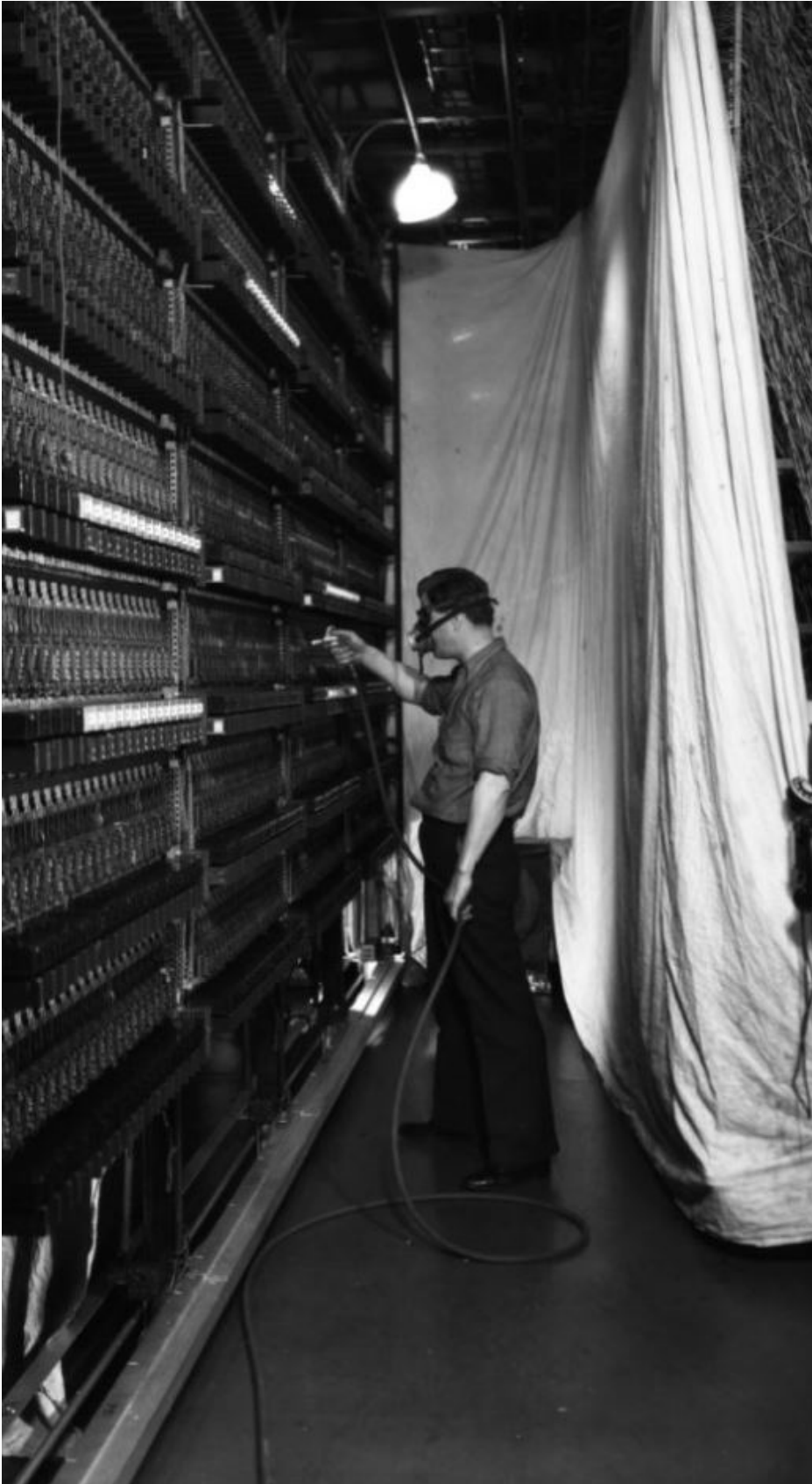
Figure 10: This photograph is included as an example of what telephone exchanges generally looked like on the interior. This photograph was NOT taken in the 12 Scott Street facility. It was taken at an unknown location and is titled, "A man air hosing off a switching board at the phone company." The switching equipment illustrated was typically installed in a Northwestern Bell Telephone Company facility such as the exchange at 12 Scott Street. The photograph also illustrates the types of interior finish materials used in the rooms where the switching equipment was typically housed. Equipment like this could have been installed in the 1947 and 1956 additions. Photographic source: Bostwick-Frohardt Collection, Owned by KM3TV and on permanent loan to The Durham Museum. Identifier BF92-1405. Dated 1936-03-12.
