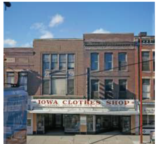
Figure 5: 536 & 538 W. Broadway prior to renovation in 1976. Courtesy of Richard Warner and Pottawattamie County Historical Society (PCHS).
