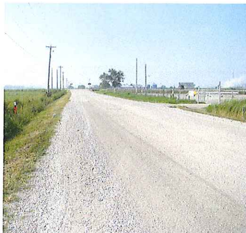
Southern view of 192nd Street.
