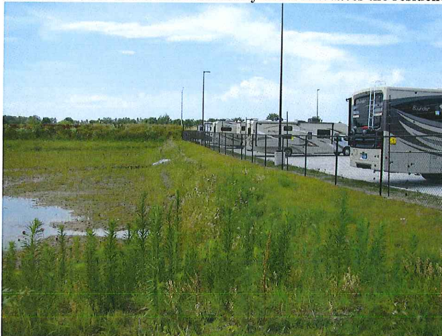
Exhibit B: View of the electric security fence that faces the residential area to the east
