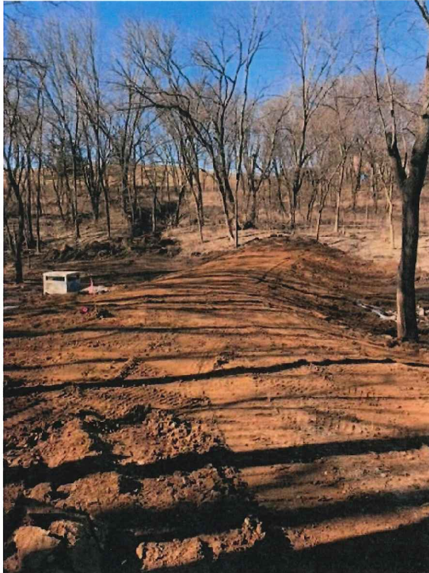
Existing Sediment & Detention Basin
