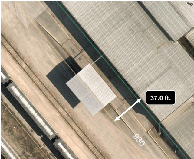
Exhibit A: Aerial photograph of the existing fill area/weigh scale on subject property
